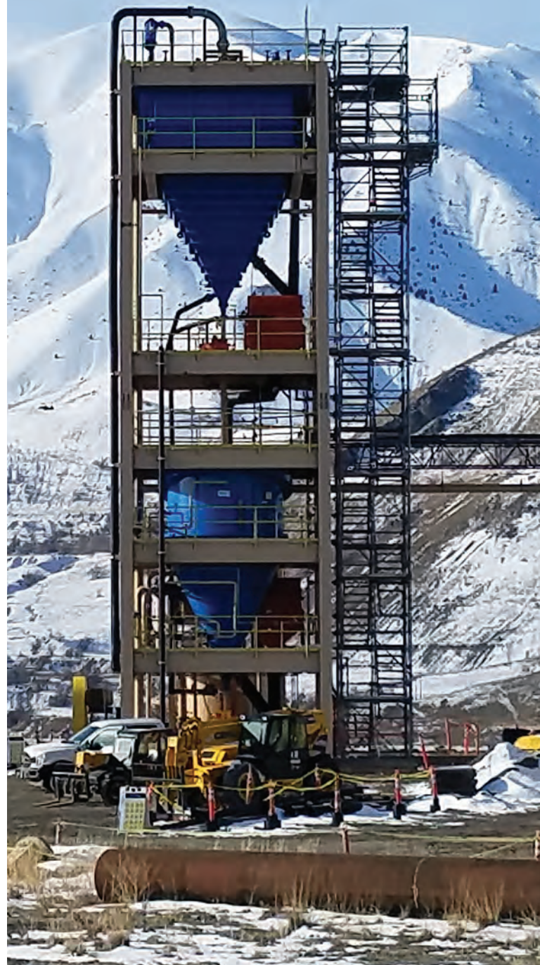
▲ HydroFloat CPF circuit for tailings scavenging at a Cu/Mo Plant.
